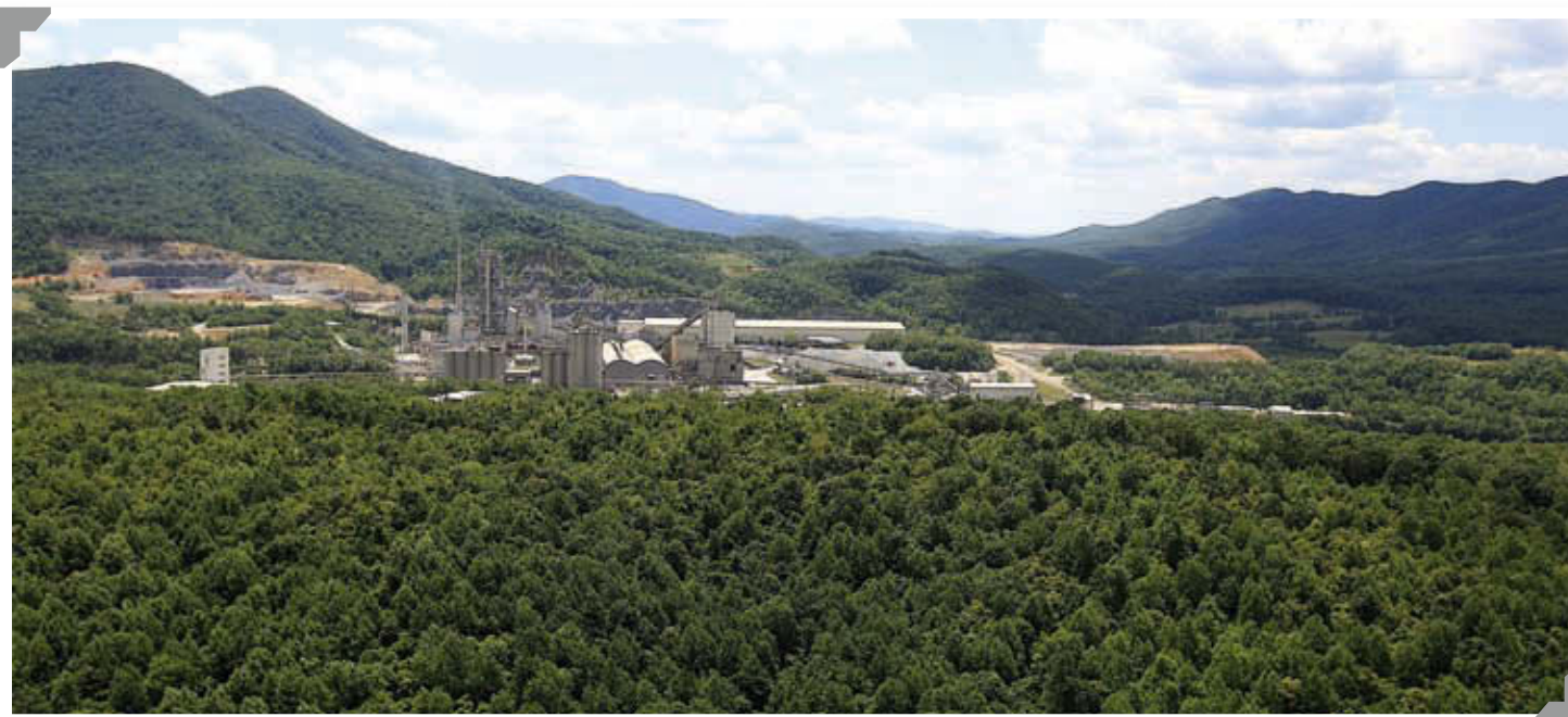
Roanoke Plant, USA
