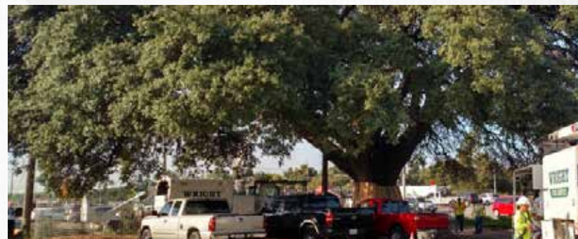
The photo shows one of the stately live oak trees with trunk armor and barricading while project work is progressing.
