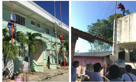
Installing a Wi-Fi access point on Cebu Island, the Philippines
