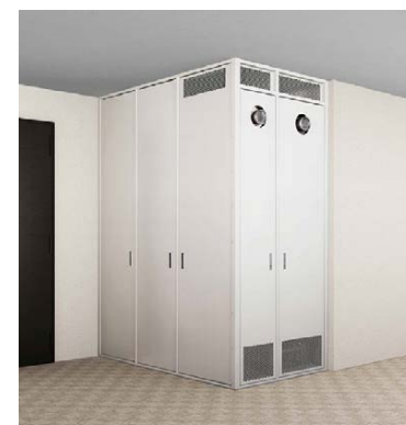
Image of a fuel cell installed inside an apartment building
