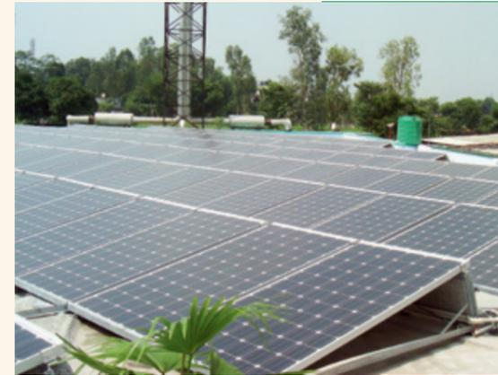
Gangaganj is a 100 KWp non-penetrating rooftop solar power plant and the first of its kind in the Indian telecom industry. This initiative has resulted in saving over 80 tons of CO2 emissions.
