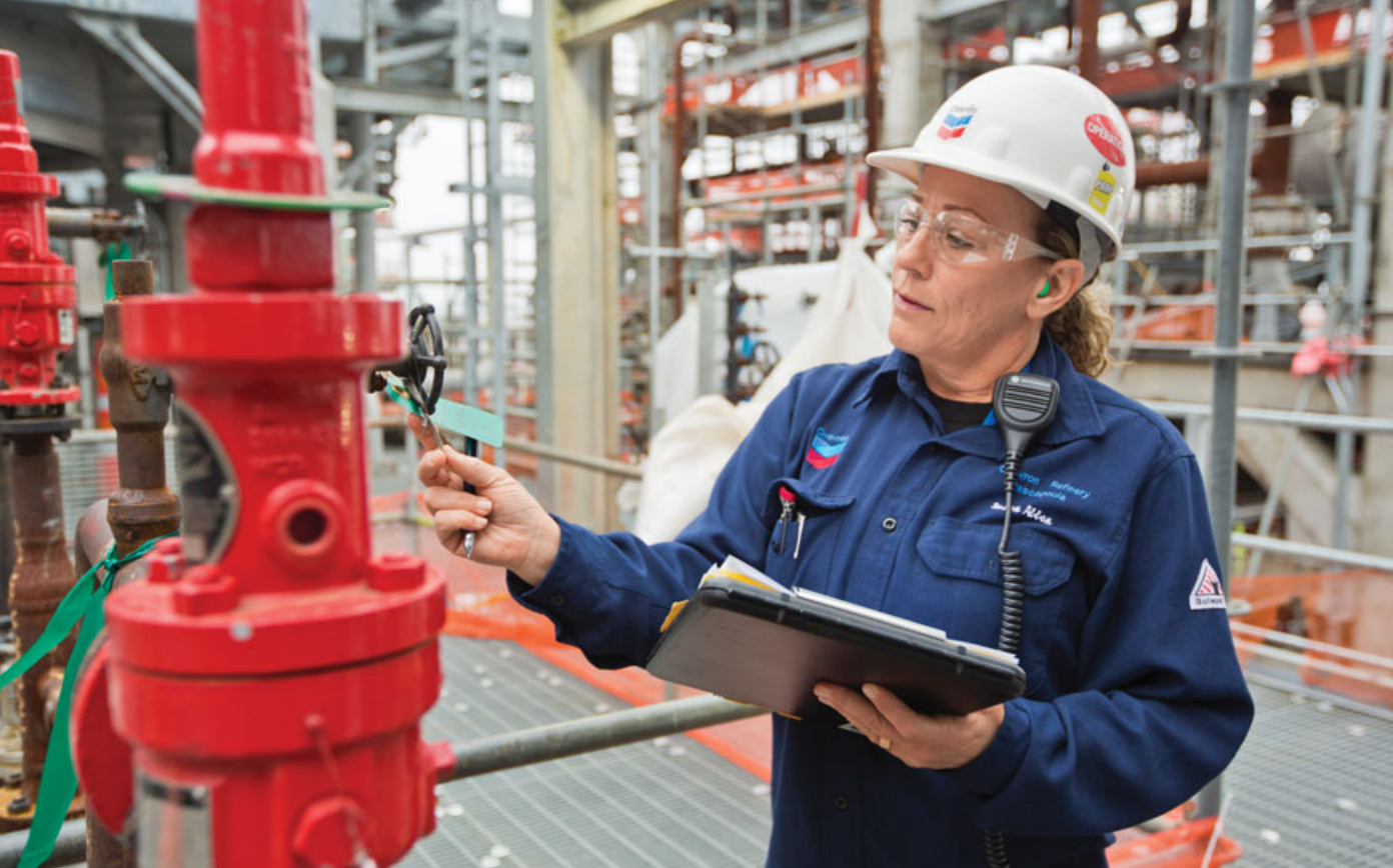
Above: Susan Allen, head operator at Chevron's Pascagoula, Mississippi, refinery, verifies that a pressure-relief device is properly tagged, dated and set correctly at the Pascagoula base oil plant, where she is on assignment as an operations representative.
