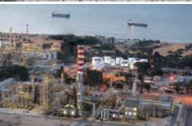
View of the refinery. At the forefront the Hydrocracker Complex (2005)
