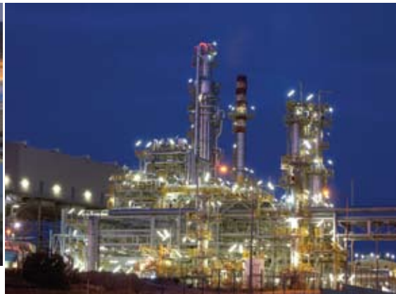
Night view of the Crude Distillation Unit (2010)
