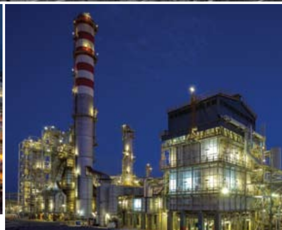
The Hydrocracker Unit by night (2005)
