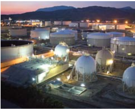
View of the LPG tank farm (2009)
