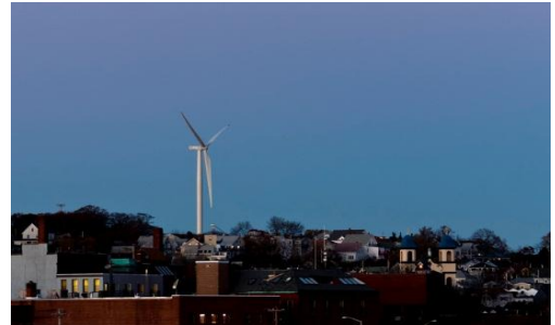
The completed 2.5 MW turbine as seen from the edge of Gloucester, MA. The turbine is mounted on a 328-foot tower and was connected to the grid in November 2012.
