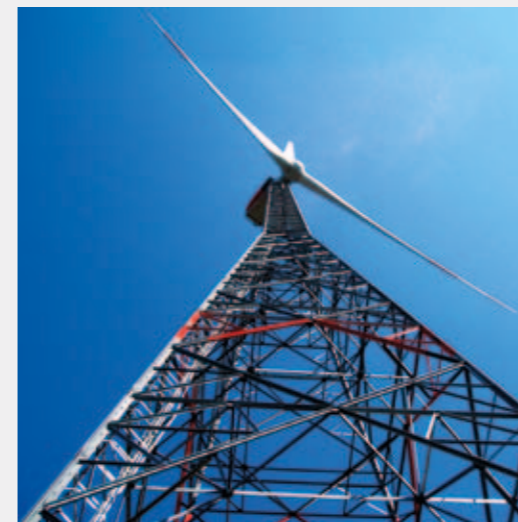
The output from a wind turbine increases significantly at taller heights. Hot rolled angles with a leg length of 300mm have been developed for use in lattice tower wind turbines, to produce 140m or 160m towers, compared to the usual 100m.
