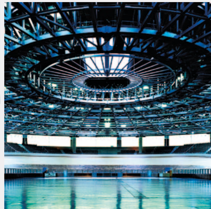
By substituting standard structural steels with high strength HSTAR®, as at the Velodrom in Berlin, the weight of steel columns and beams for buildings and other physical structures is reduced by about 30%.
