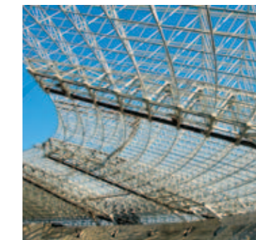
An example of an application of the HISTAR® beams, Baku stadium, Azerbaijan.
