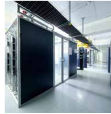
Deutsche Börse uses Equinix, a data centre offering best standards in ecofriendly IT
