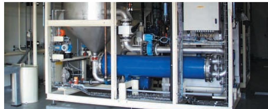
Wastewater evaporator in Vénissieux, France
