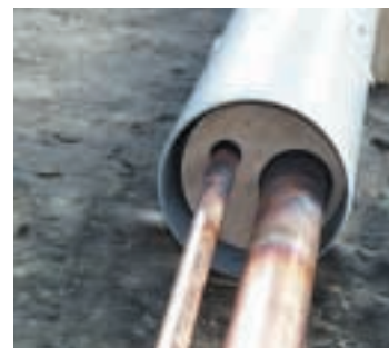
Tube-in-tube arrangement prevents soil contamination in Tilburg, Netherlands.
