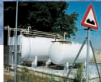
In Alcalá de Henares, Spain, we have decommissioned subterranean oil tanks, replacing them with above-ground tanks for better control.
