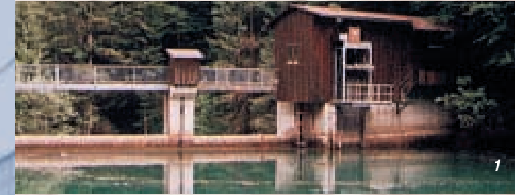
Photo 1: At Blaichach in Germany, our own hydroelectric plant supplies about 60% of our electric energy.
